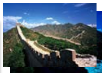
TO100-328 The Great Wall of China
