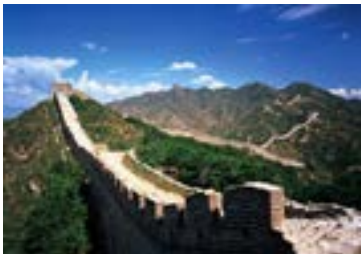
TO400-006 The Great Wall of China
